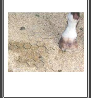
**Porous pavers** are manufactured in a variety of designs and materials. Concrete turfblock for grass paving began in the mid-1940's and plastic versions were invented in the late 70's and early 80's. Porous pavers are generally a cellular grid system filled with dirt, sand, or gravel.
