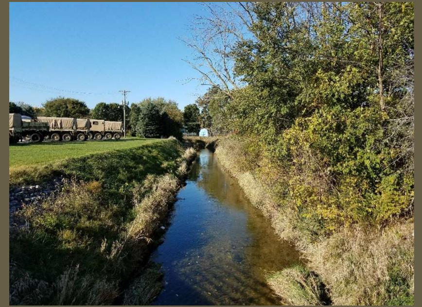
Downstream from E. Fordice Street. The entire Fordice to East Street reach has been armored with gabions. The left bank in the foreground shows the development of a small bench. Vegetation on the left bank is minimal. The right bank is steeper and more protected by the extensive woody vegetation.
