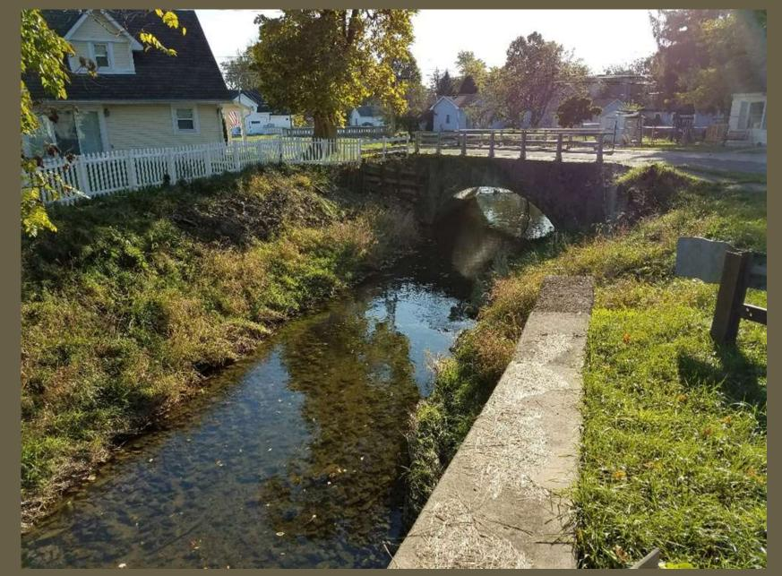
Looking downstream from Busby Street to Jameson. Reach is armored with concrete blocks, poured concrete walls, rubble, large blocks, and wood pallets.
