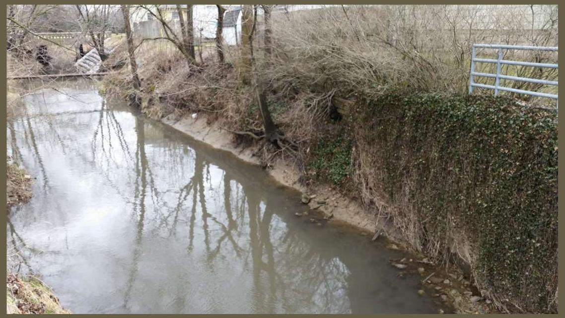
Left bank looking upstream from the Meridian Street Bridge. The scour line is visible along the left bank. Note the gabion baskets at the upstream end.
