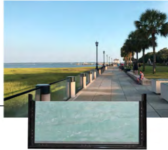
Glass Flood Wall
