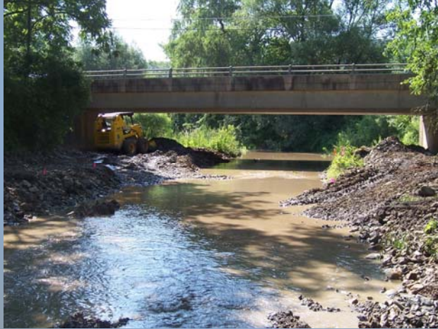
Start of Construction June, 2007
